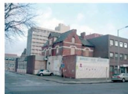
View 4 Existing building South East corner
