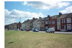
The houses on Queen Street front the existing Leisure Centre, and the project provides the opportunity to create a buffer that will improve their outlook and provide space for parking.
