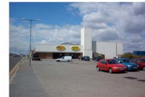
The Enterprise West building is in need of a significant investment that will be enabled by the project, and with Redcar Beach recognised as a world class Kite Surfing location it is ideally sited to take full advantage of the beach, acting as the focus for a wide range of Lifestyle sports.
