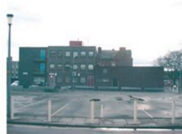
View 2 Existing building across university car park
