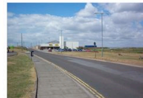
Looking east along Majuba Road, this illustration shows how Majuba Road bisects the site, and presents no obstacles to prevent traffic building up speed.
