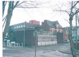
View 1 Existing building South West corner
